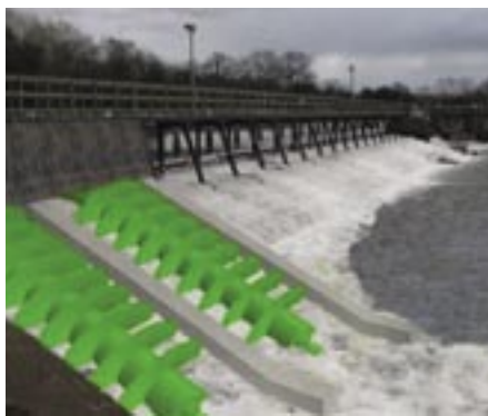
An indicative representation of the turbines – Ham Hydro plans to install 4 screws on a different section of the weir
